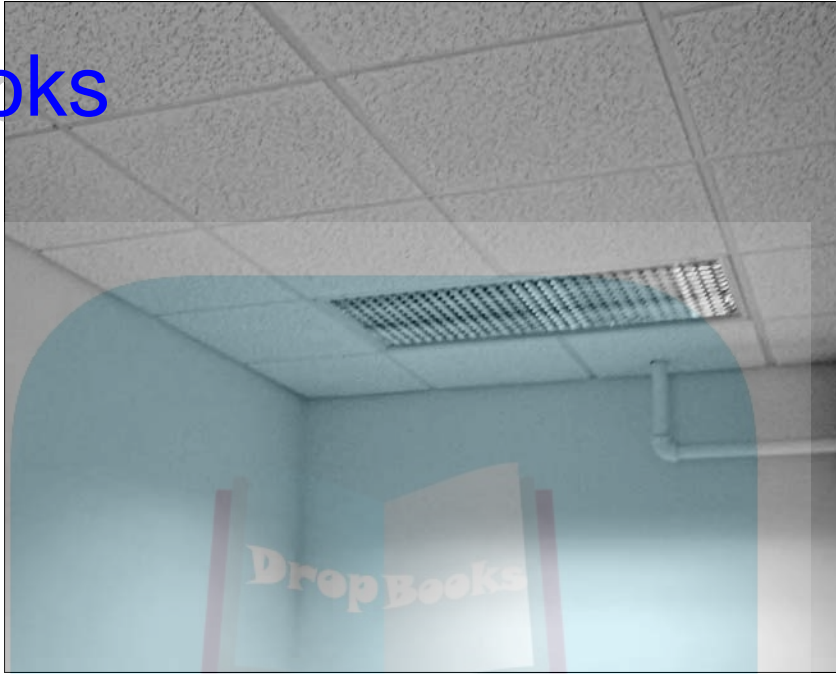
Figure 10-2: Parabolic louvered lenses allow you to use fluorescent lights in many kinds of rooms.
